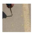
Use high speed power drill with 1/2" masonry bit and core drill each hole 5" in
