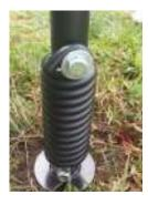
Insert the post into the other end of the spring and attach them using the remaining hardware in the spring kit.
