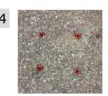
Make sure top of mungo plug is flush with asphalt surface.
