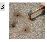
Using the wide flat hammer stuff mungo plugs into core drilled holes.
